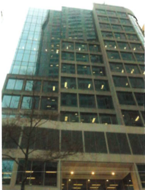
Photo 1: The Building located on the site.
