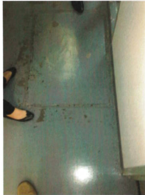
Photo 12: The surface of the ground level with a sealed hatch.
