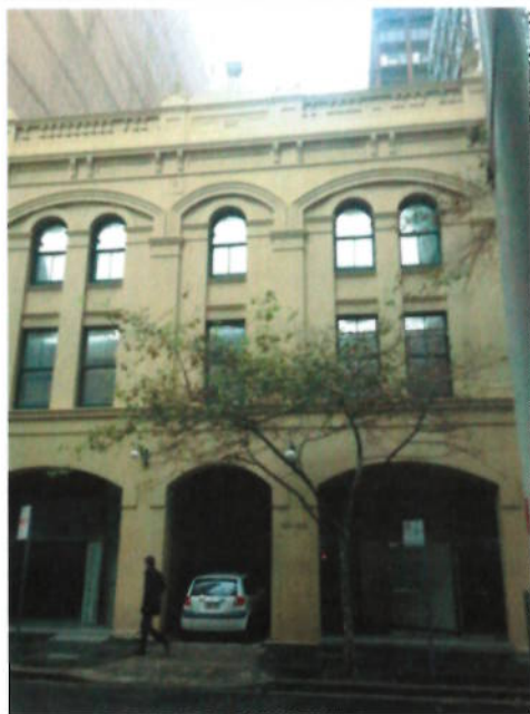
Photo 3: Heritage building located to the north of the site.
