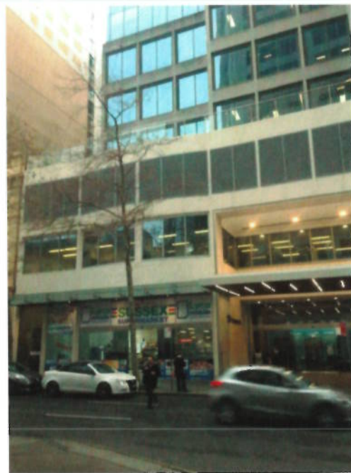
Photo 2: The supermarket located within the north-western corner of the site.
